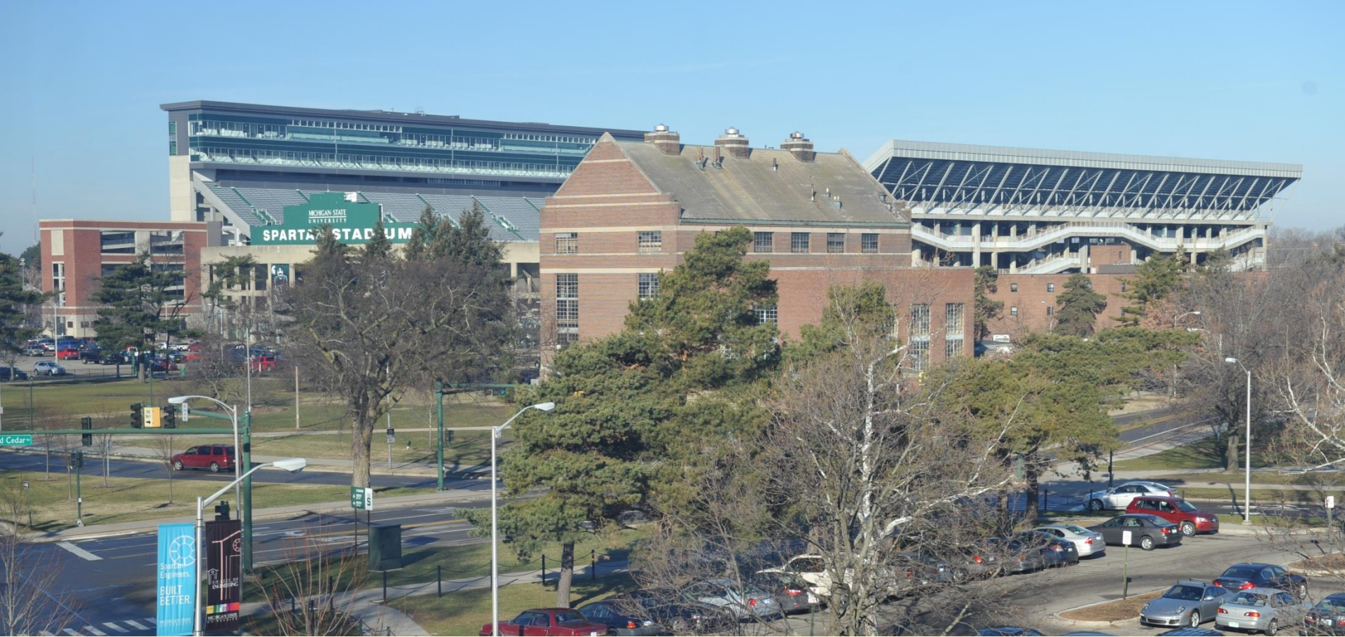
Capstone Lab View of Spartan Stadium sans Smokestack
